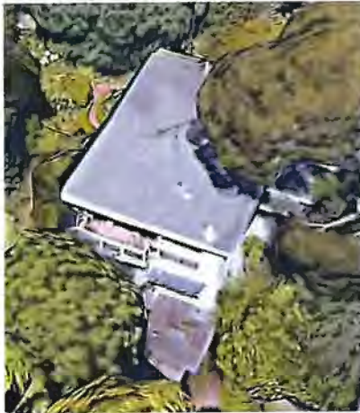
2c. 3(?)-story, 6-unit, hillside site not visible from street. WFTS: Hillside cripple wall assumed based on similar buildings.
