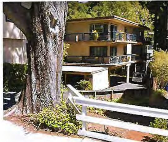
2d. 3-story, 4-unit building on rear of lot. WFTS: Open first story assumed based on partial visibility from street.
