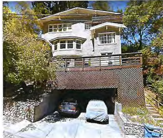
2b. 3-story, 4-unit, hillside site. WFTS: Hillside cripple wall assumed based on age of building and partial height retaining wall at right side.
