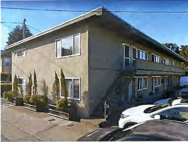
1a. 2-story, 12-unit. No WFTS; first and second story units align. All parking is outside the building.
