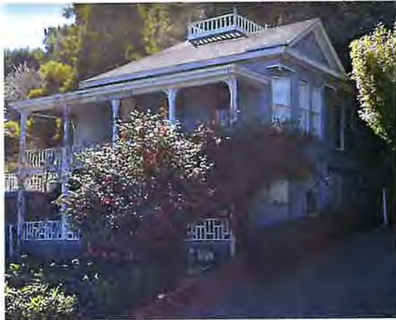
2a. 2-story, 3-unit, sloped site. WFTS: Cripple wall assumed based on age of building and elevation of first floor relative to grade.
