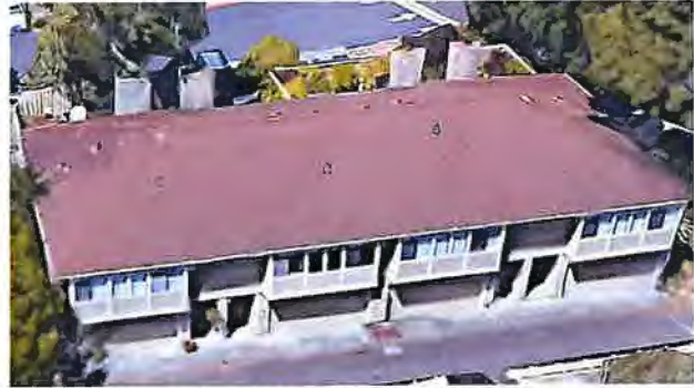
1d. 2-story, 4-unit townhouse. WFTS: Long side open to accommodate ground story parking.
