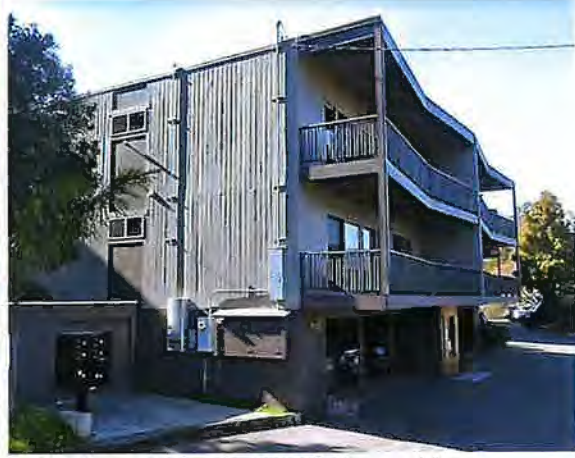
1b. 3-story, 4-unit. WFTS: Long side open, to accommodate ground story parking.
