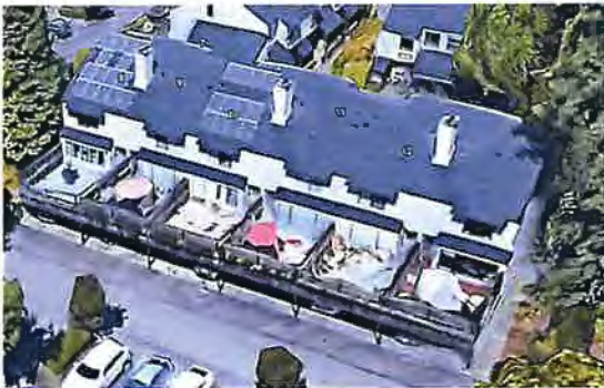
1c. 3-story, 6-unit townhouse. No WFTS. Parking under deck looks like "long side open" WFTS but is outside the building and is structurally similar to an attached carport.
