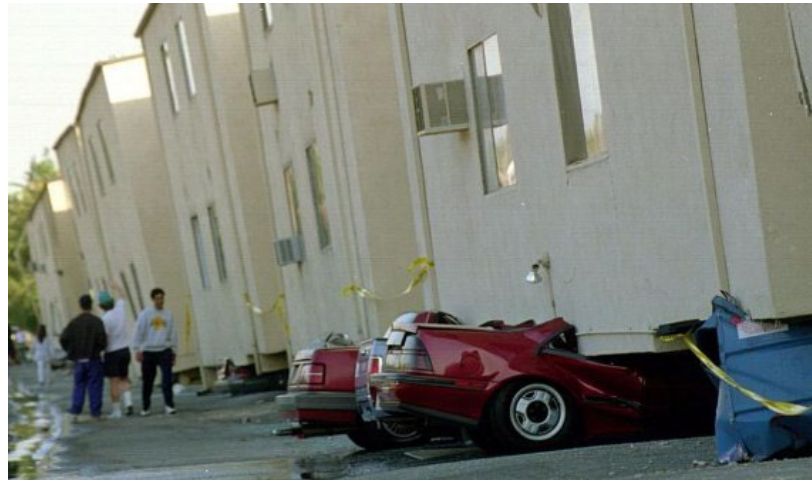
Collapsed 3-story building, Los Angeles, 1994 Northridge earthquake (photo: Boris Yaro, Los Angeles Times)
