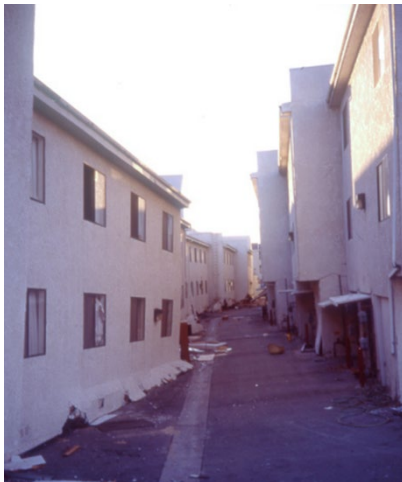
Collapsed and near-collapse 3-story buildings, Los Angeles, 1994 Northridge earthquake (photo: Gary D. Avey)
