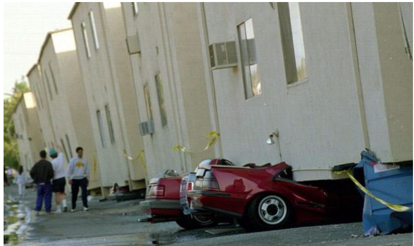
Collapsed 3-story building, Los Angeles, 1994 Northridge earthquake (photo: Boris Yaro, Los Angeles Times)
